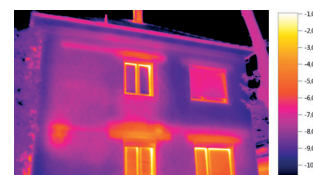
Thermal image with ScaleAssist
