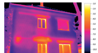
Thermal image with ScaleAssist
